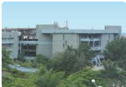
College of Engineering, Pune
